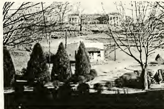
THE BUFFALO STORE looks lonesome sitting at the foot of the hill beneath Sutton Hall, doesn't it?
