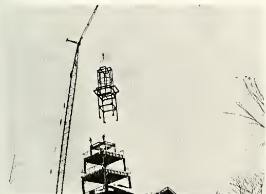
STEEPLE RAISING -- The cone of the steeple was placed in position yesterday on the W. R. Walker Memorial Chapel, on the Milligan College campus. This section of the steeple is 32 feet in length and weighs 9,755 pounds.
