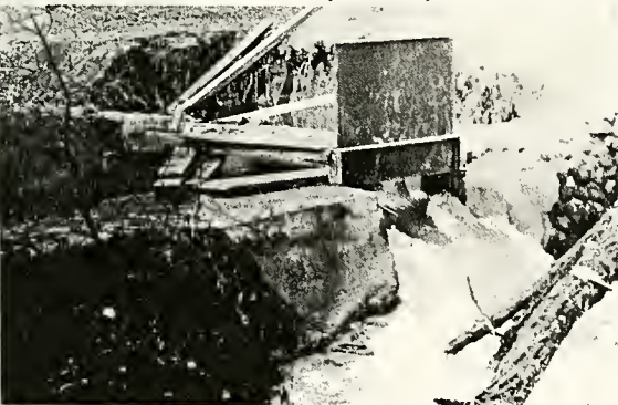
The traditional beauty of the Buffalo Creek dam will soon be restored as the new flood gate is now in place.
