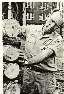
Preston Kite and crew are expertly reconstructing "Old Fort Watauga" in preparation for the May Day Pageant.
