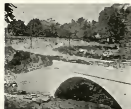
CONGESTION MINIMIZED--Construction on the new state highway is being maintained.
