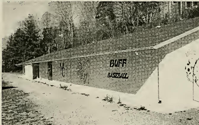
The still unfinished athletic building adjacent to Anglin Field. Photo by Mark Amstutz.
