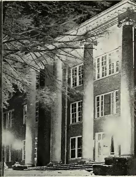
Left: Administration Building
