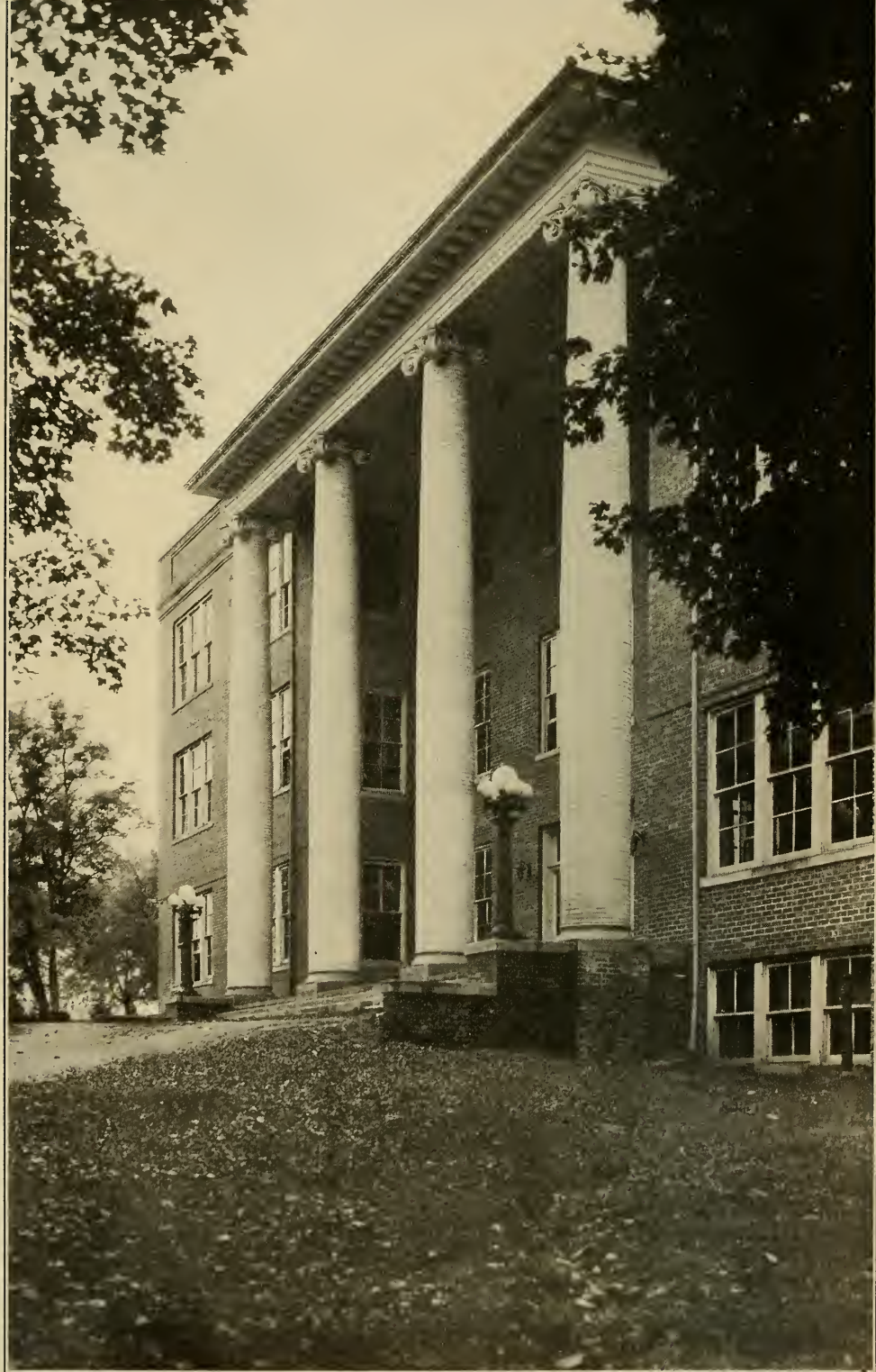
ADMINISTRATION BUILDING (FRONT VIEW)
