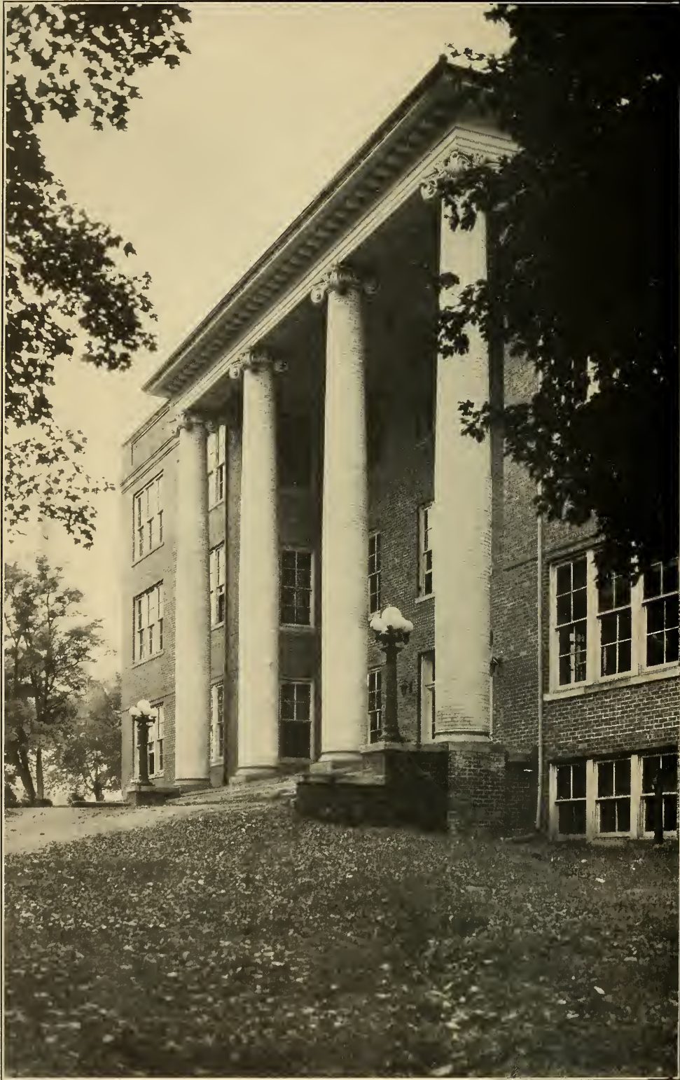
ADMINISTRATION BUILDING (FRONT VIEW)
