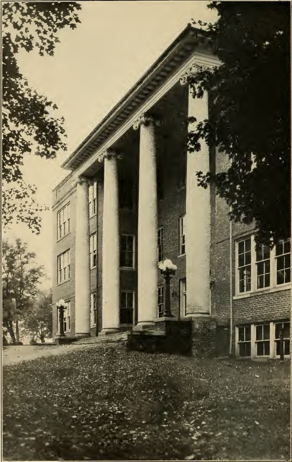
ADMINISTRATION BUILDING (FRONT VIEW)
