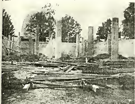
SCIENCE BUILDING GOES UP--In a break with the tradition established by the Milligan Bridge, construction is actually progressing on the new science building.
