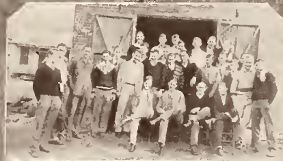
Power House Club
