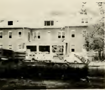
Hardin Hall under renovation
