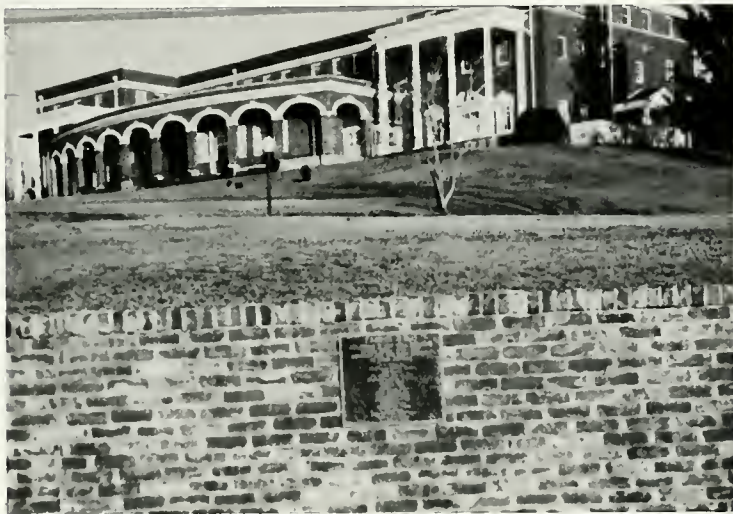
The Pardee wall is all that remains after the destruction of the dorm in 1992.
