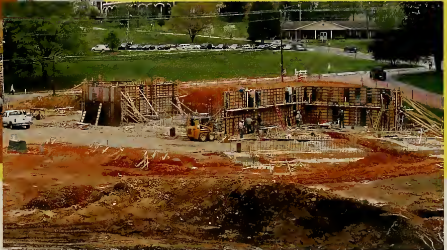
CONSTRUCTION AS OF 04/20/06 -->
