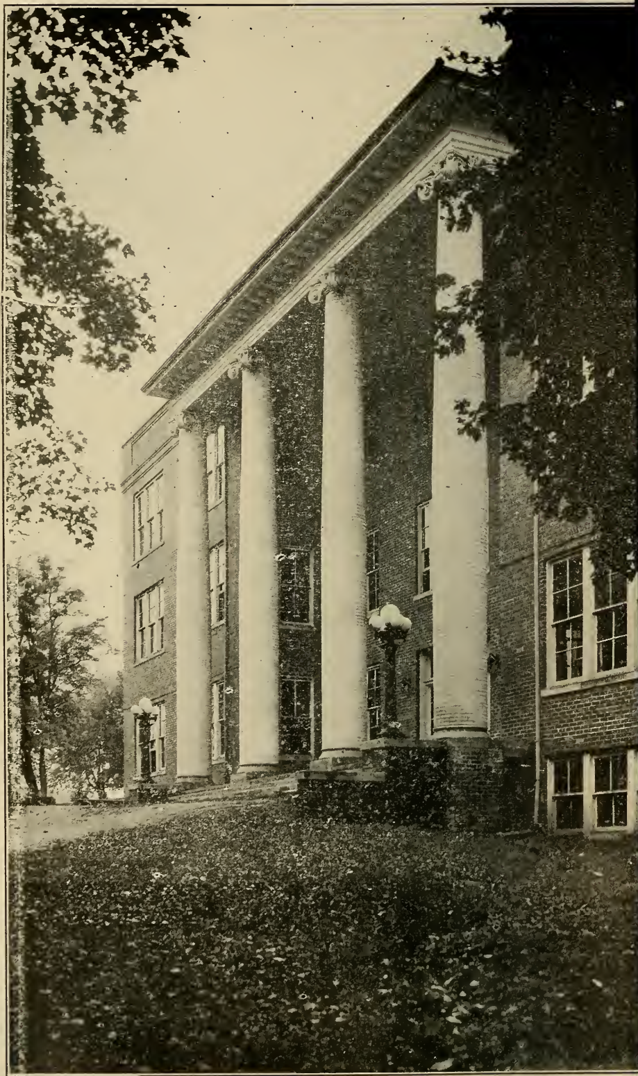
ADMINISTRATION BUILDING (East View)
