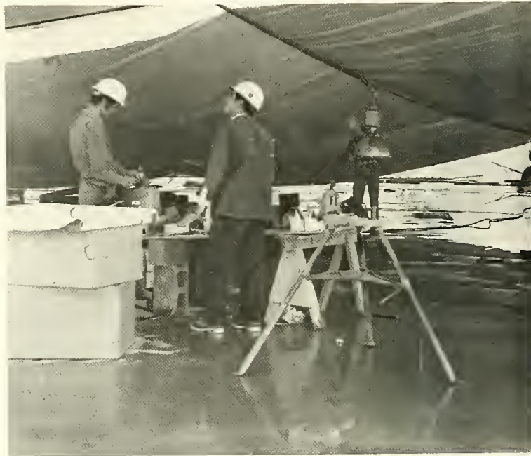
Workers prepare to blow-up fieldhouse roof.
