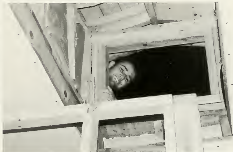
Up on the roof top, reindeer, Nope Zach Pearson. Come down through the chimney, not through the window, that is if your 'Santa Clause'. This part of the home looks just about finished.
