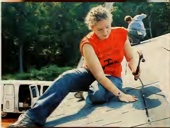
Valerie Palich snaps a chalk string on the roof of the house they are building so the shingles are straight.
