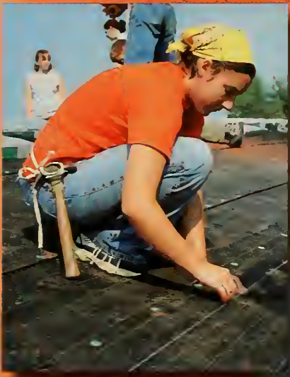
Valerie Palich snaps a chalk string on the roof of the house they are building so the shingles are straight.
