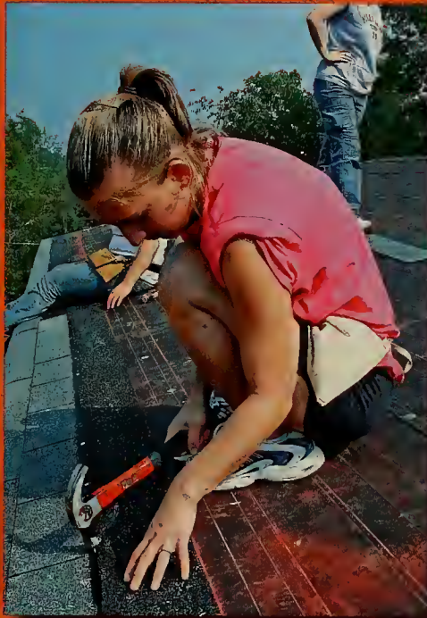
(Below Left) The hammer meets the nail as Mackenzie Whittington shingles the roof.
