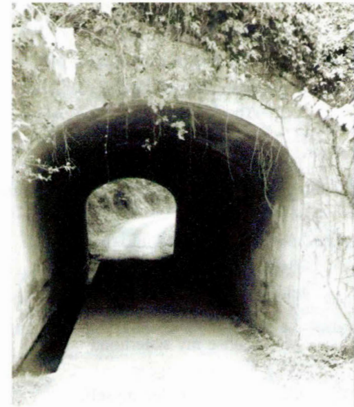
"Phipps Bend Tunnel"
